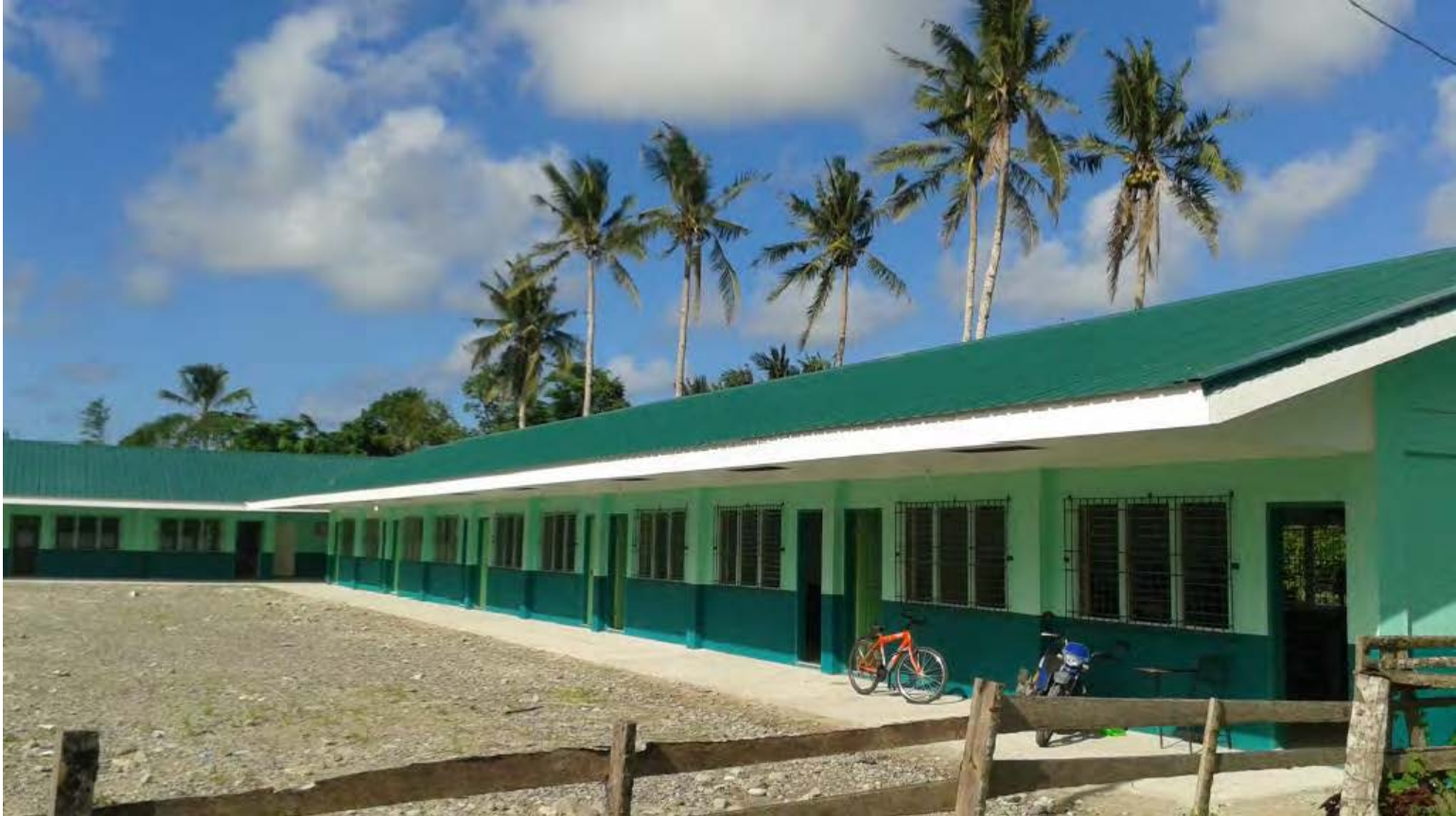
9-classroom building for Manlilisid National High School in Javier, Leyte
